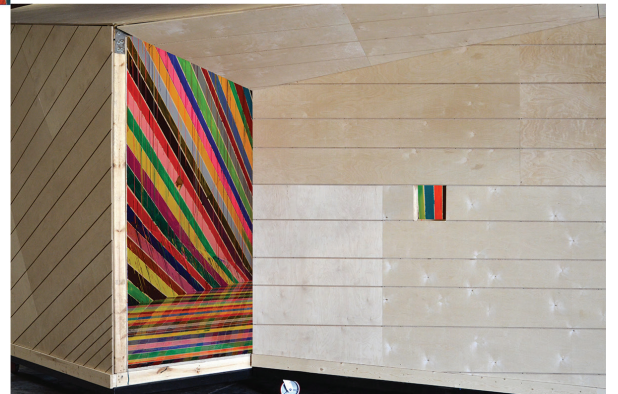
Where two volumes slip past each other, entry ways are created, with small punctured windows which fall between lines of the engraved pattern.
